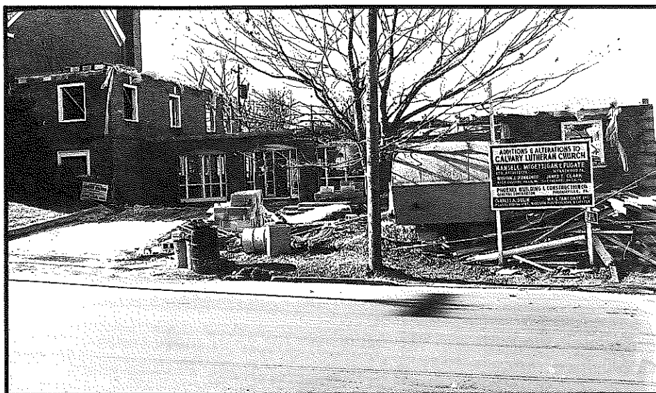
Construction begins in 1966 on the Education Wing
